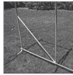
Structural wind brace on each side
